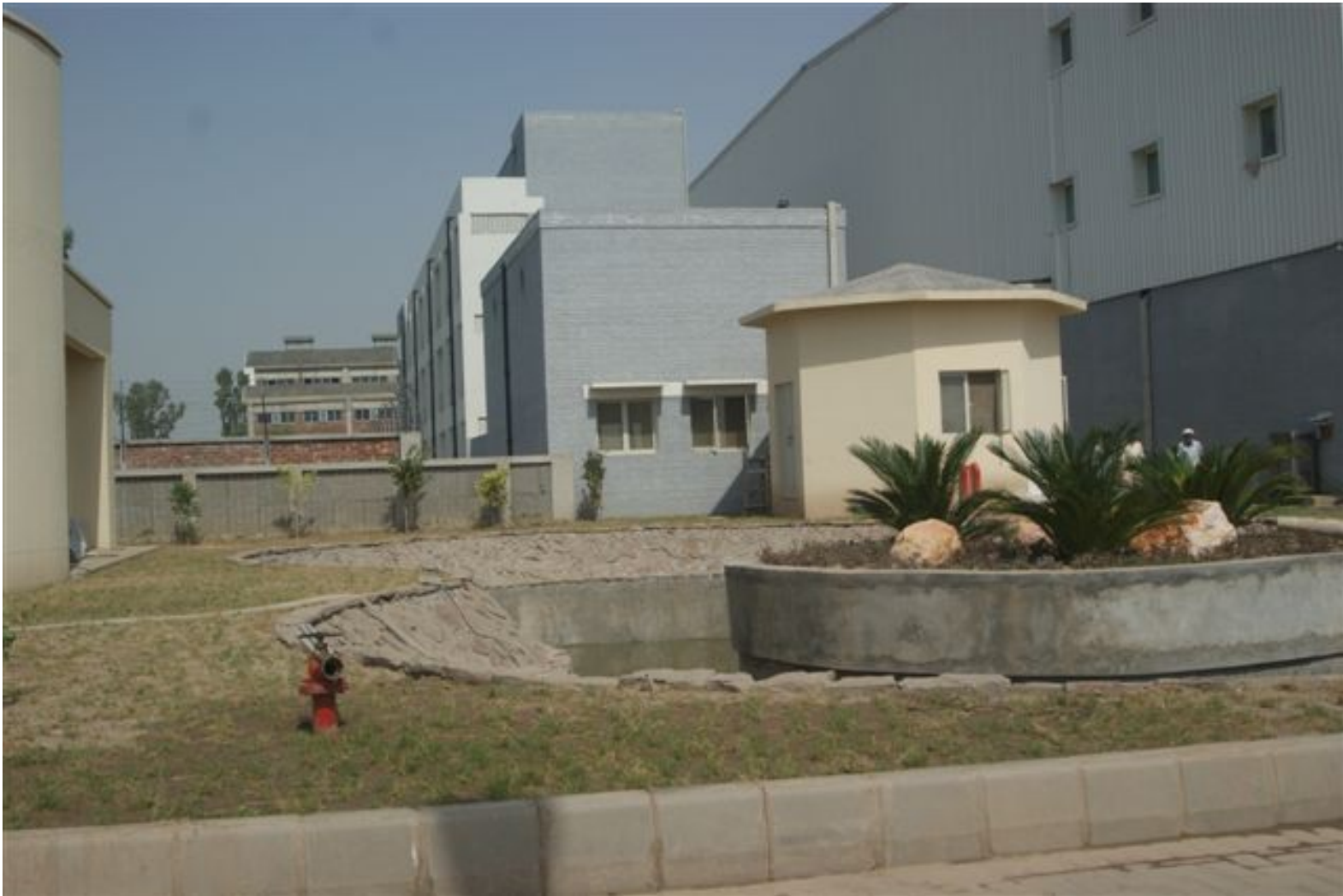
View of Turbine room, Battery room, Workers' Accommodation & Water reservoir
