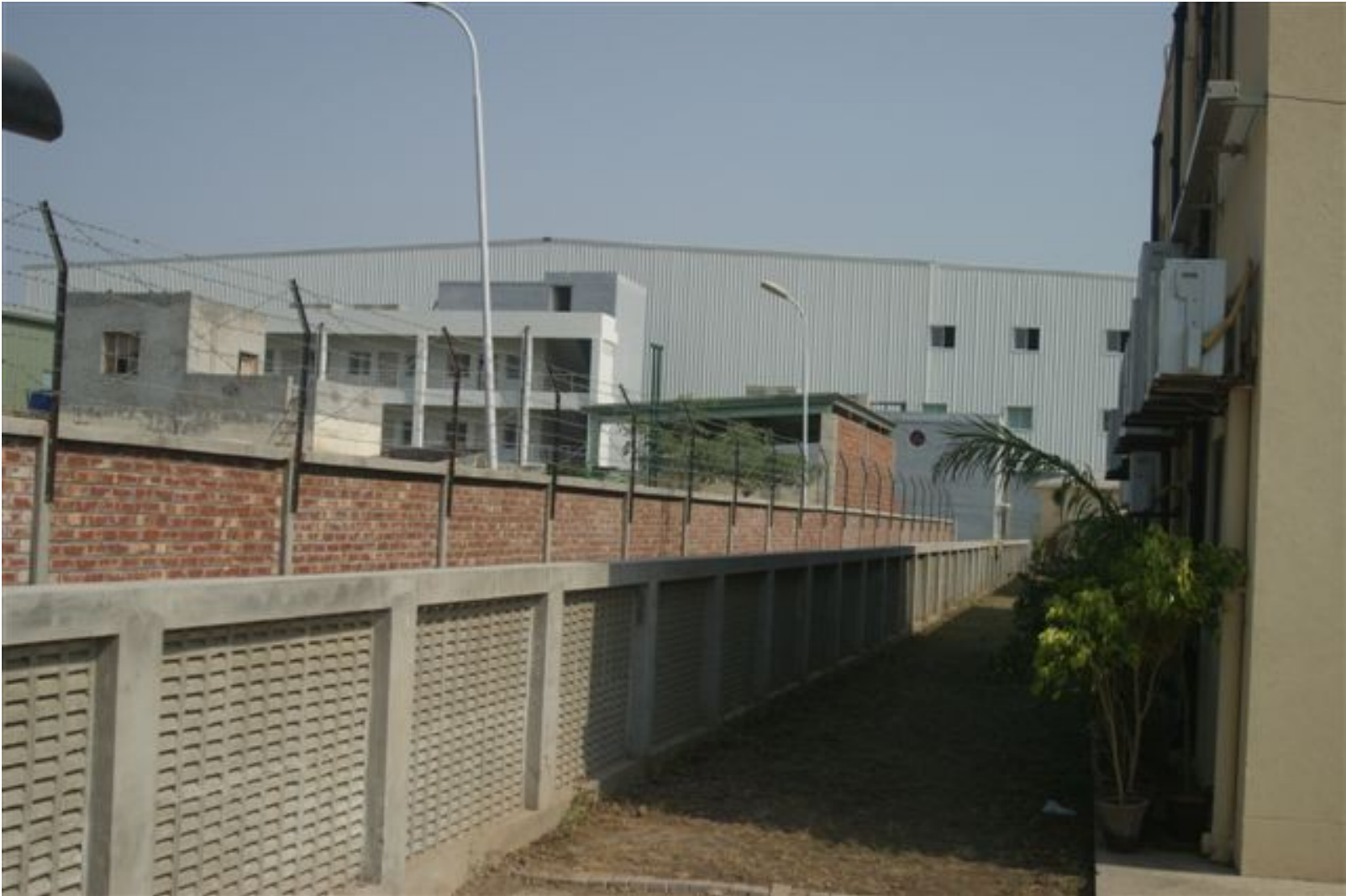
Office Block Back side
