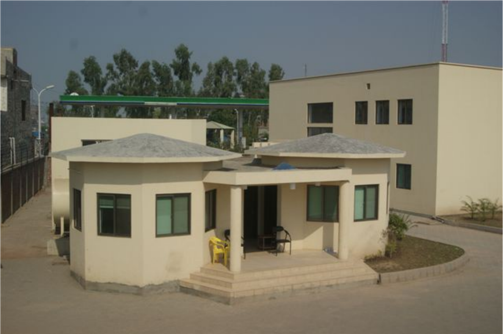
Main Gate – Office
