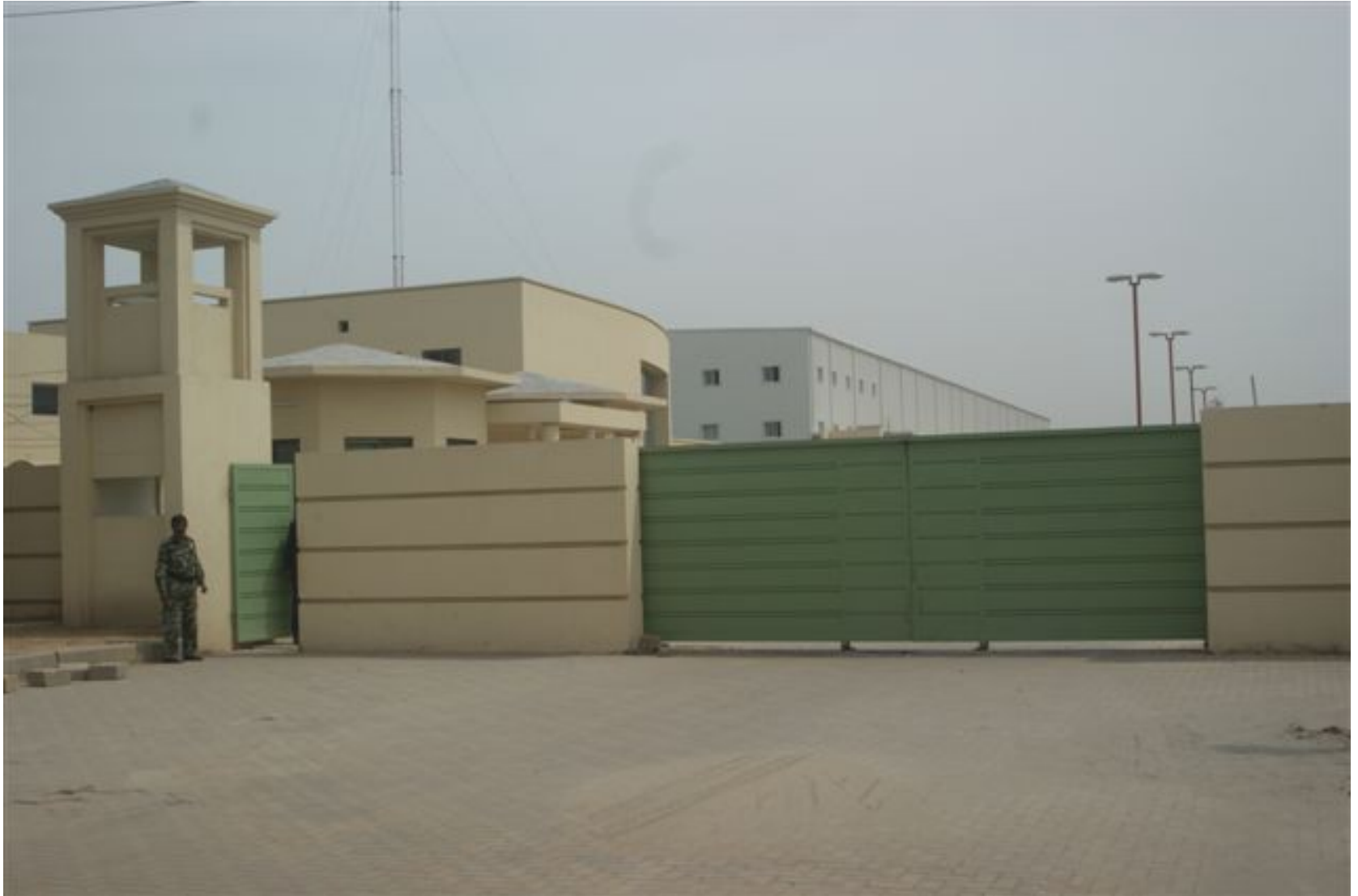
Main Gate – External View
